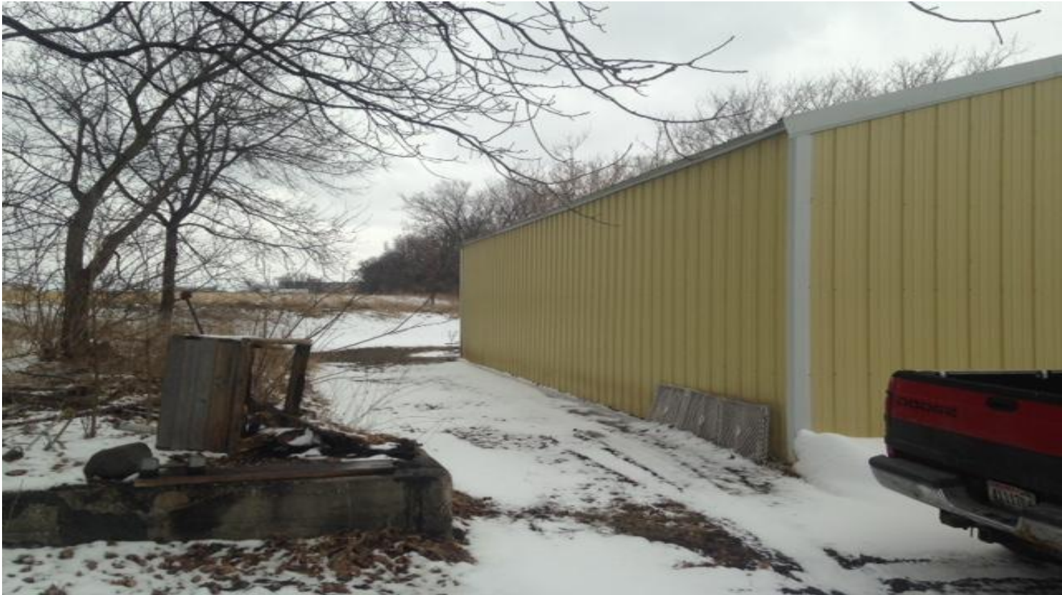
Exterior of Shop/Storage Garage
